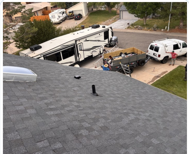
COMPLETED ROOF FIELD
