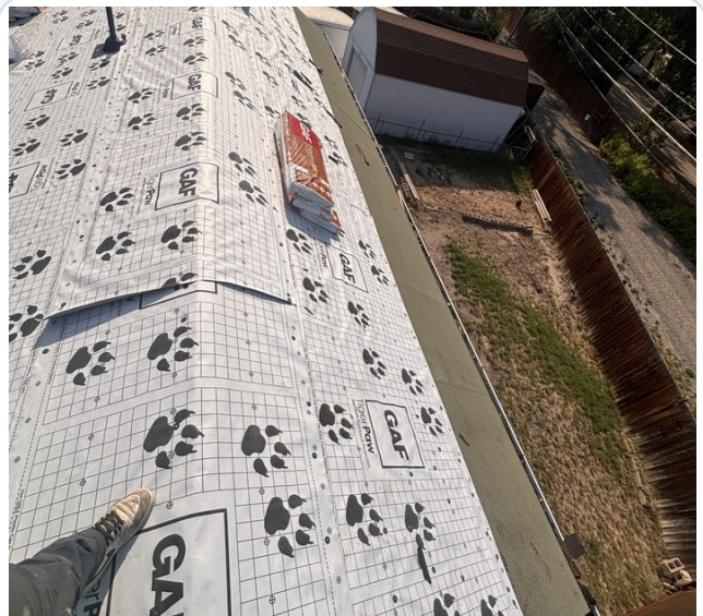
PROTECTED ROOF DECK
