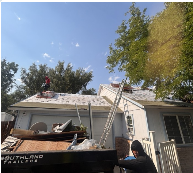
ROOF REPLACEMENT PREPARATION
