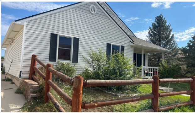
SIDING PROJECT - BEFORE
