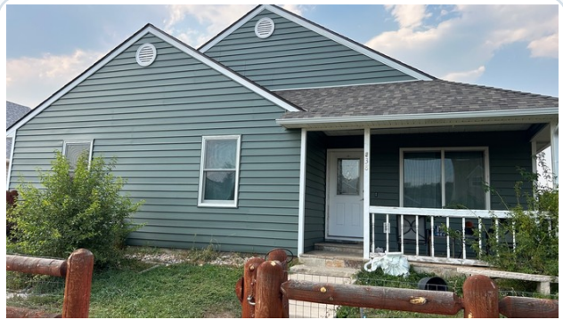
SIDING PROJECT - AFTER
