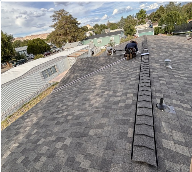
RIDGE-CAP INSTALLATION
