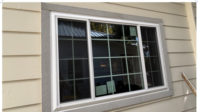
COMPLETED WINDOW INSTALLATION
