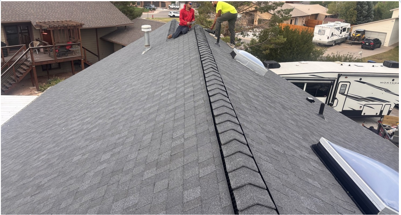
COMPLETED RIDGE AND SHINGLE INSTALLATION
